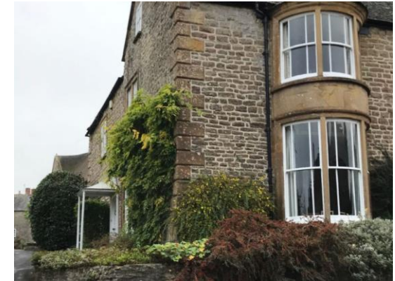
Photo: Junction of Queen Street with the High Street, Yetminster, showing corner treatment with windows on both sides
