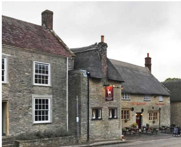
Photo: Yetminster High Street showing varying rooflines
